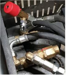
fit the <u>STEAM VALVE for HOT BOX OUTLET line - C1.510HBKIT</u>. <u>This must always be open</u>, and must be fitted to the temperature line, as this will prevent a high temperature explosion which can result in serious or fatal injury.
